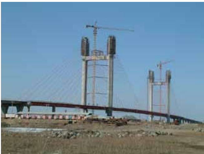
Cable stay bridge
