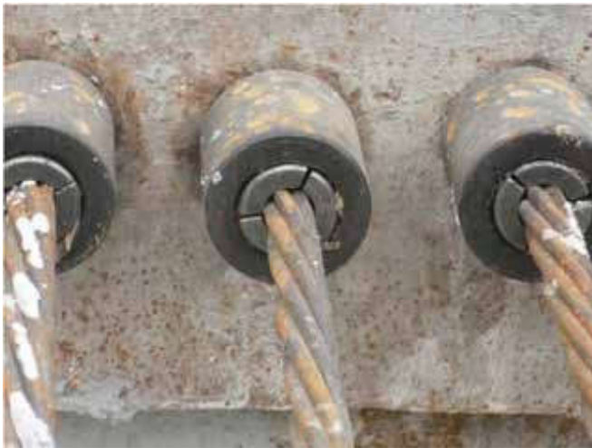
CPS Post-tensioning construction
