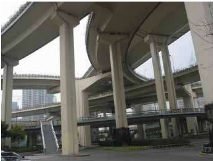
Elevated ring roads
