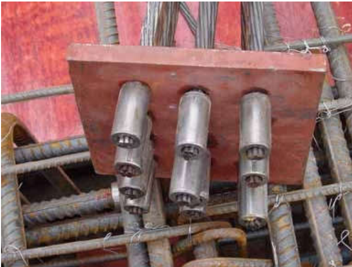
Fixed P anchorage at Construction site
