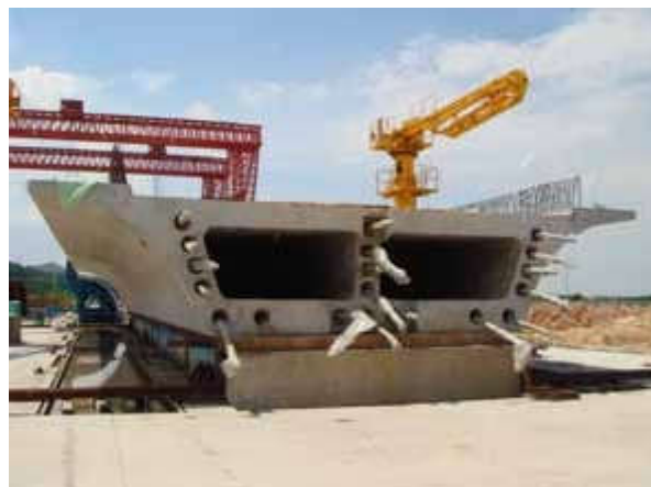
Post-tensioning on box girder
