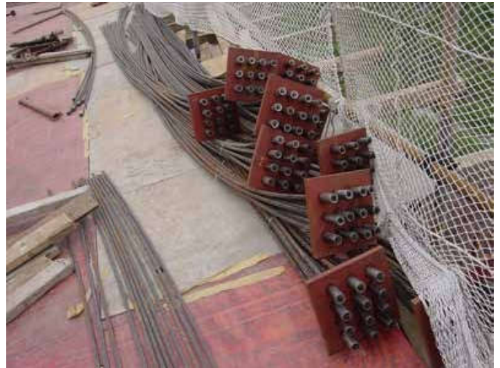
Fixed P anchorage at Construction site
